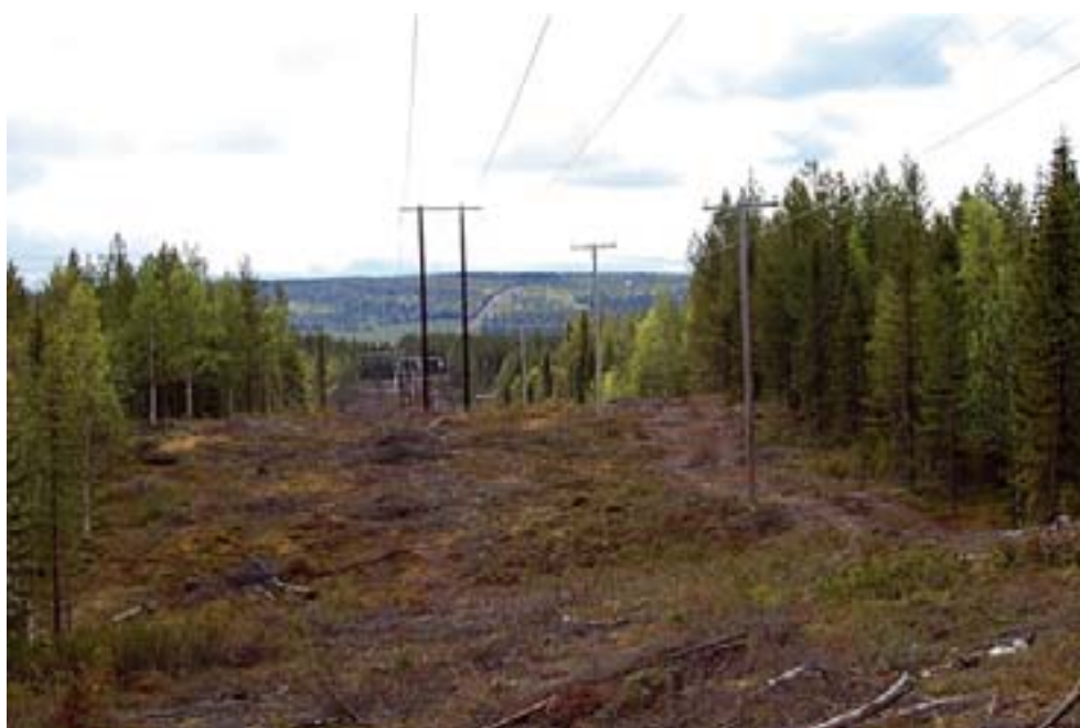
New power line at Jokkmokkliden wind farm in northern Sweden. Another new power line, for Storliden wind farm, is visible in the background. Photo: Anna Skarin.
